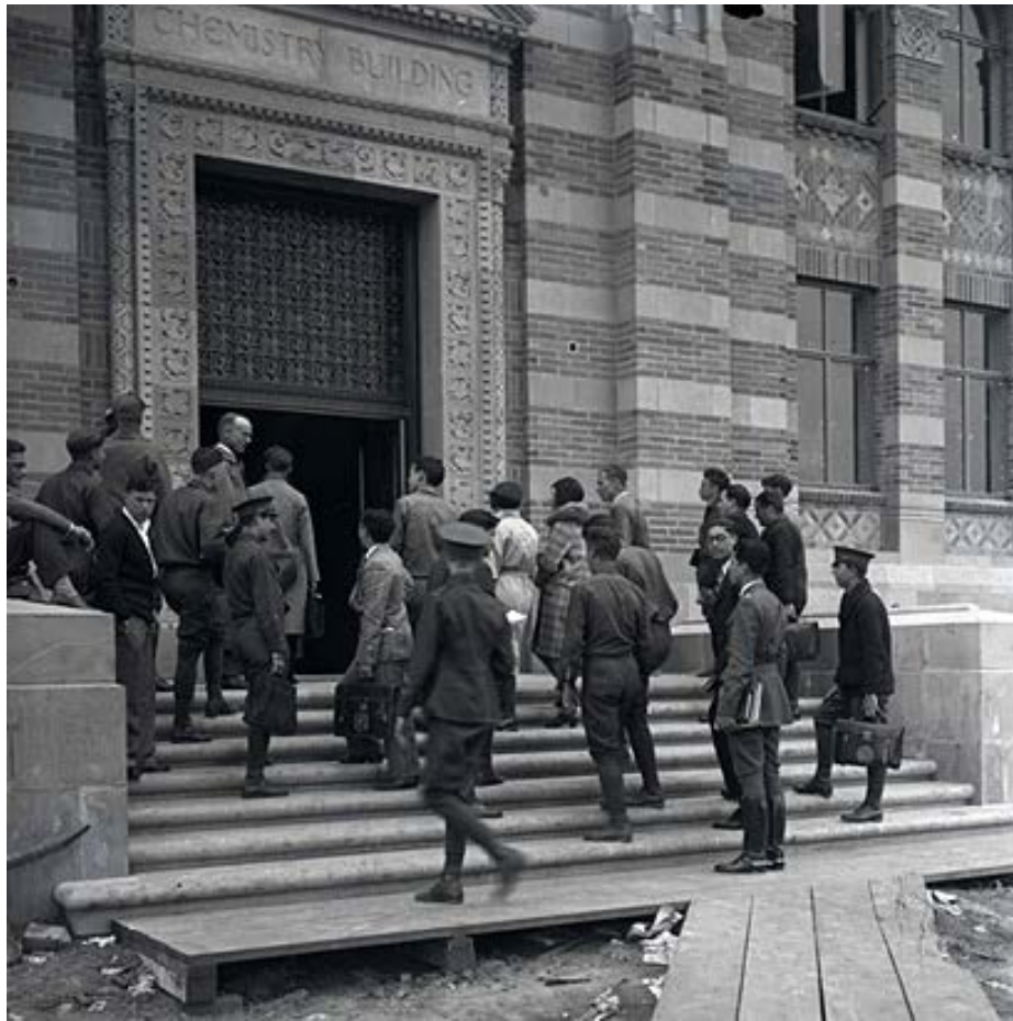
Chemistry Department building is now Haines Hall
